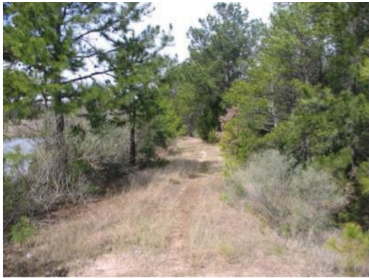
This fish pond dam likely will have problems with leakage (if not already) and breakage if the trees are not killed or removed.
