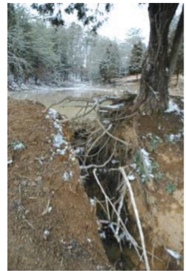
Tree roots can cause dams to fracture, leak, and eventually break.
