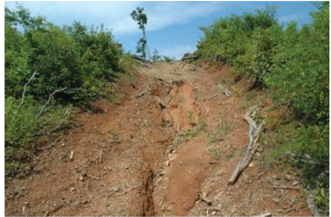
Forest roads should not be constructed perpendicular to slope. Roads such as this should be closed and planted to trees or shrubs.
